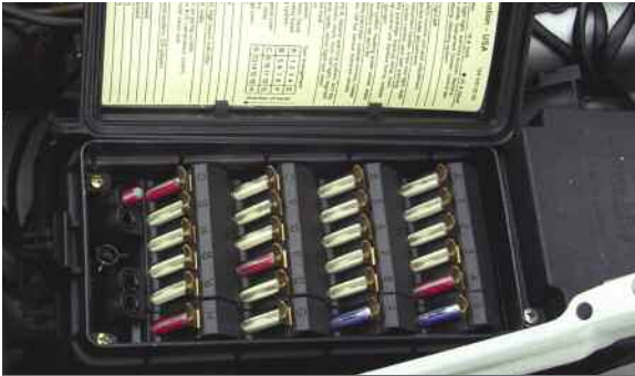
The fuse and relay box for most Mercedes-Benz cars is on the driver's side in the engine compartment, sealed with spring clips. Fuses and relays are clearly identified by position and number; voltage and continuity measurements are convenient.
