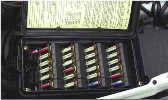
The fuse and relay box for most Mercedes-Benz cars is on the driver's side in the engine compartment, sealed with spring clips. Fuses and relays are clearly identified by position and number; voltage and continuity measurements are convenient.
