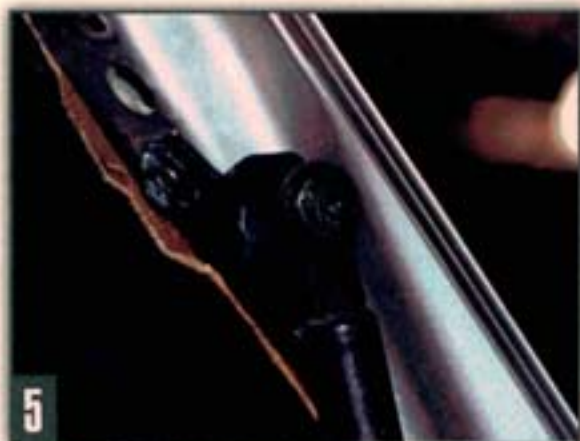
5 All we need is a little more space, right? Removing the bolts from the hood struts and repositioning them will give you a lot more room for that cherry-picker arm.
