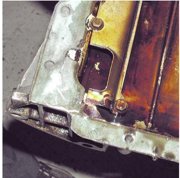
The old gasket failed right at the parting surface between the block and the rear cover. Proper positioning and the judicious use of seam sealer can reduce the chance of that happening to your work.
