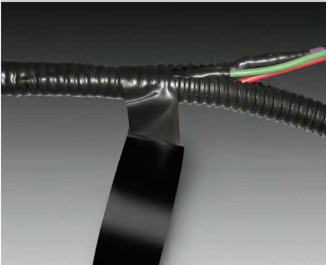
Use flex conduit to protect wiring
