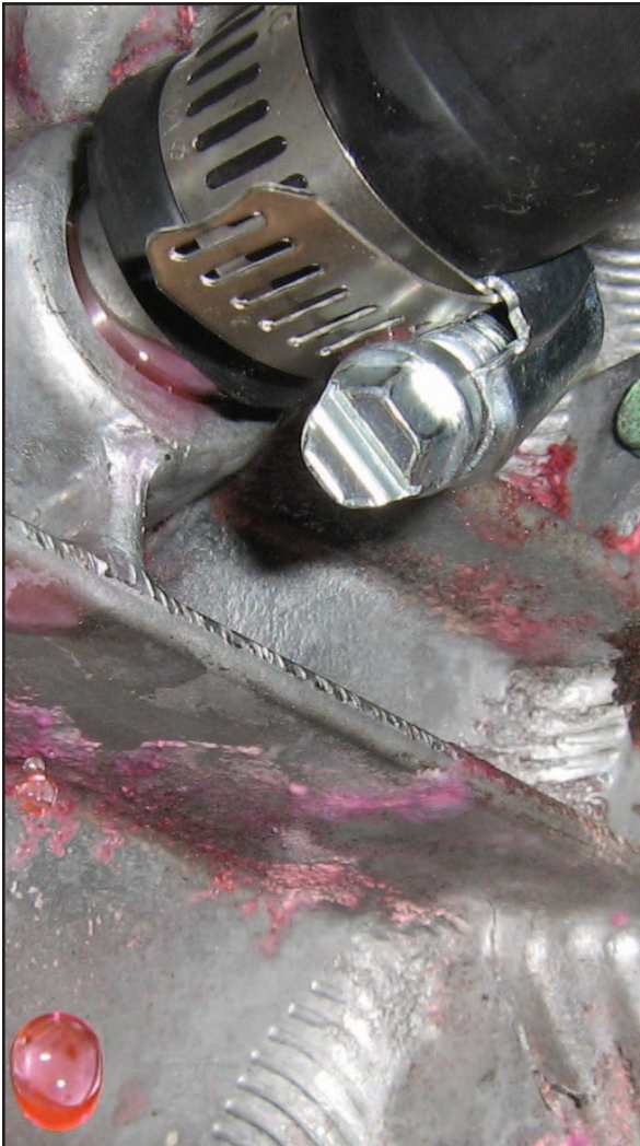
A new hose clamp won't fix this one.
