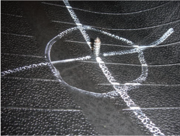
Mark the area to be repaired to avoid “losing” the injury.
