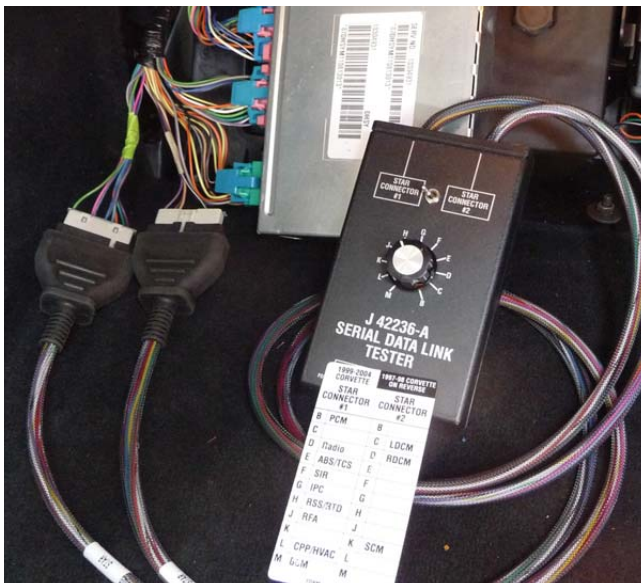
Figure 5: Removed the star connector combs from the connectors and installed the Kent Moore tool.
