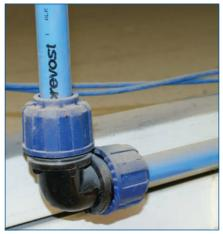
In order to prevent rust contamination as your equipment gets older it's necessary to install aluminum, plastic, or copper piping from you filtration system to your paint booths.
