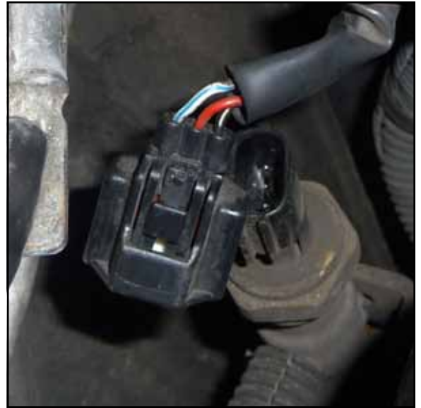
Figure 10: P/S Pressure Switch unplugged.
