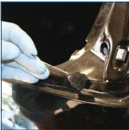
Thoroughly clean and prep the metal frame area of the vehicle before applying the primer.
