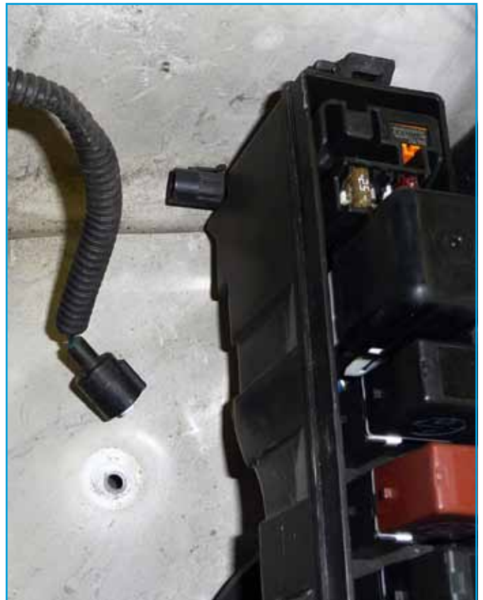
Figure 10: Open O2 heater circuit under the battery tray.
