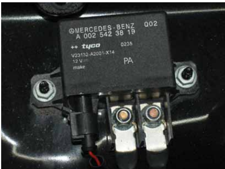
At the base of the windshield under a protective cover is the auxiliary relay. This connects the auxiliary batter to the system either to supply voltage or receive charging current for the auxiliary battery.
