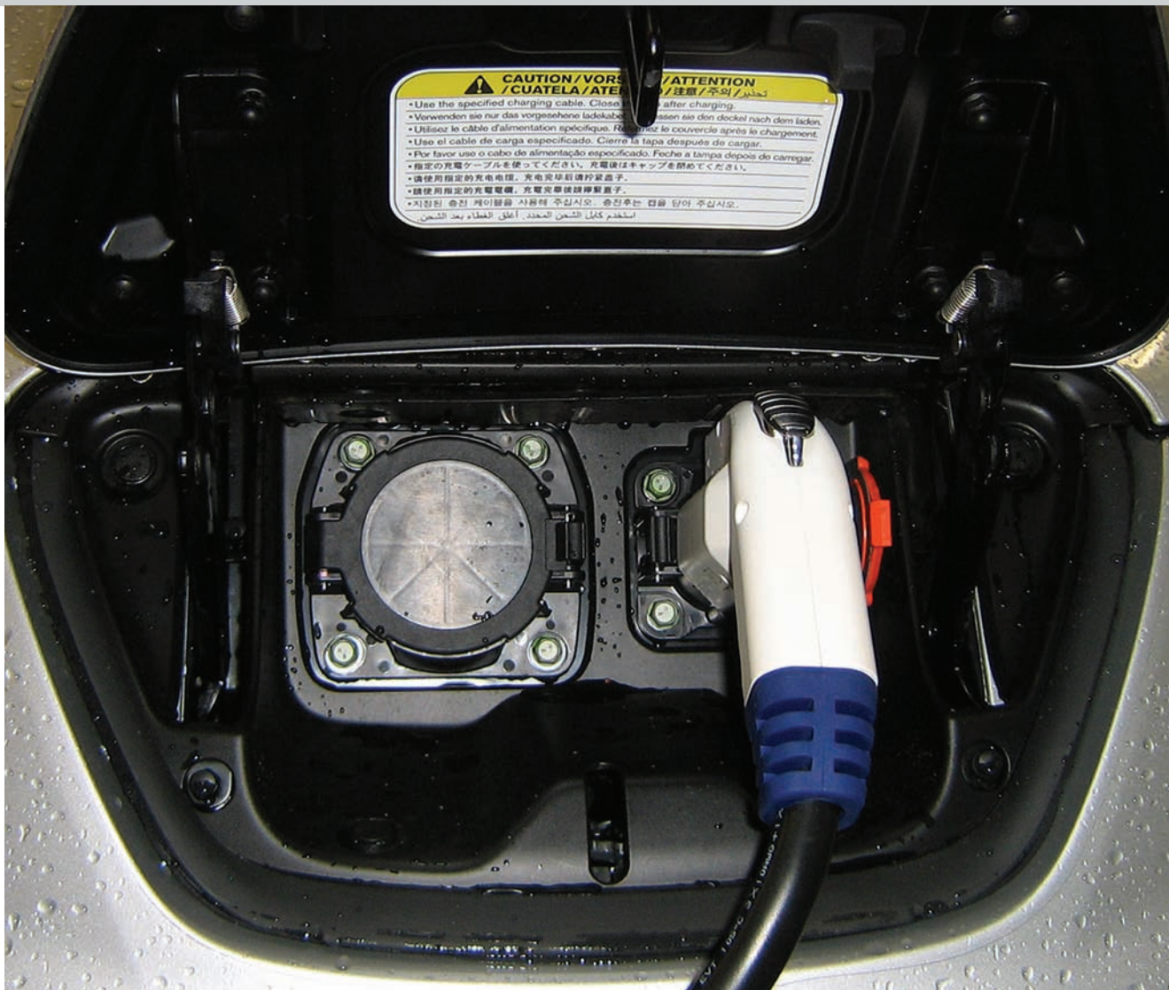
The port on the left is for quick charge. Shown here, the LEAF is using the shop's 240V to get a little charge while in for service.
