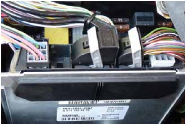
This ME Control Unit is located in the left front fuse box. When the fuse box lid is not securely fastened, it can allow water to get in. Pull the connectors and check for evidence of H2O.
