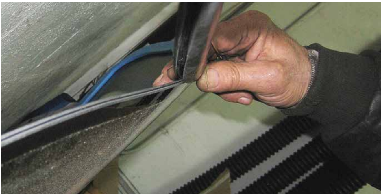
Sliding the glass into the molding channel is easy. Of course, there's a lot of prep not shown in this picture.
