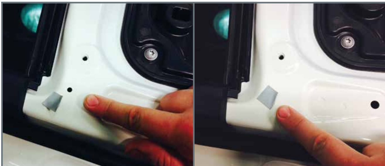
To ensure that the air pressure sensor mounted in the door cavity can register an increase in pressure that occurs in the event of a side impact collision, every opening must be sealed. Sealing tape was applied at the factory to this small hole in this M-Class SUV rear door, and must be replaced if removed during a door repair.
