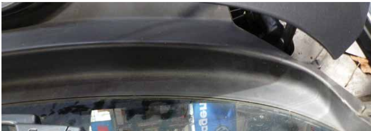
The cowl seal is very important in keeping water out of the vehicle as well. These seals can become damaged or pop out of their guide track occasionally. If these seals are not fully seated, rain water can wash directly down the windshield into the air intake. Not good!
