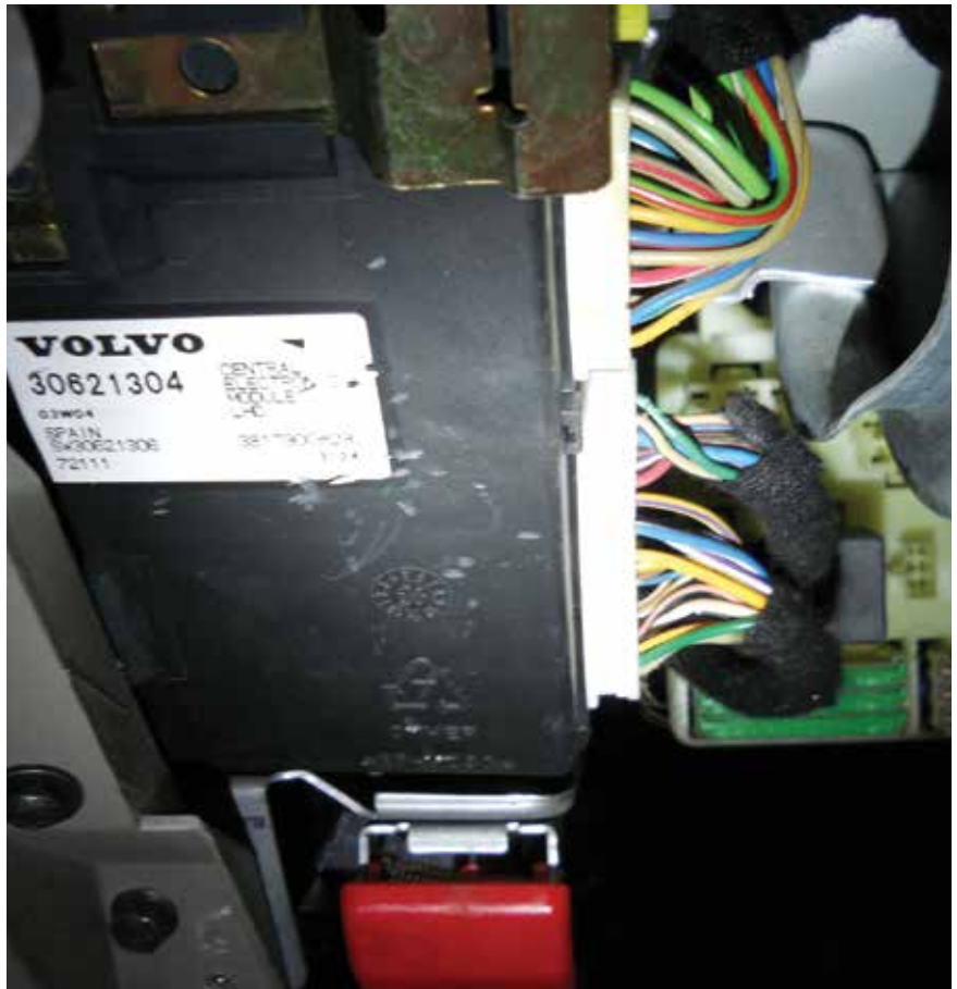
The Central Electronic Module completes the circuit to the low beams.
