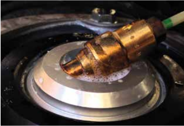
The leak here is revealed by the bubbles on the top of the air strut.
