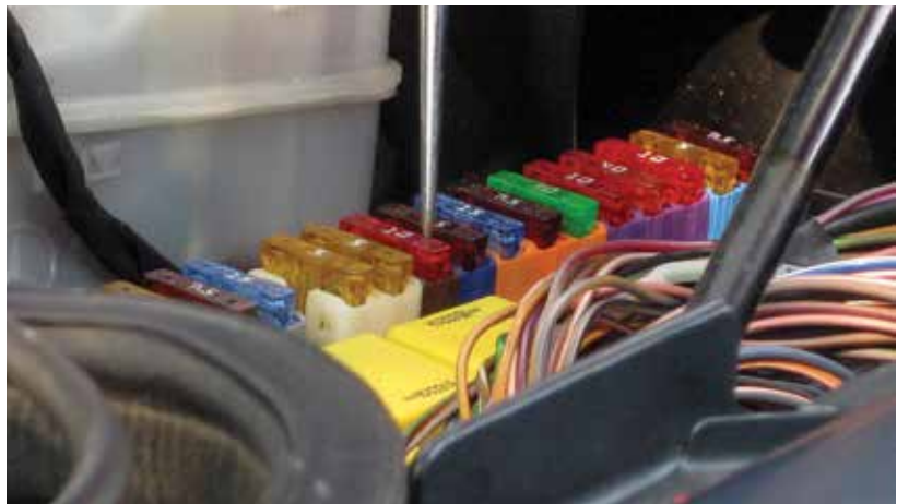
If you want to check fuses or any feed of battery voltage with a test light...
