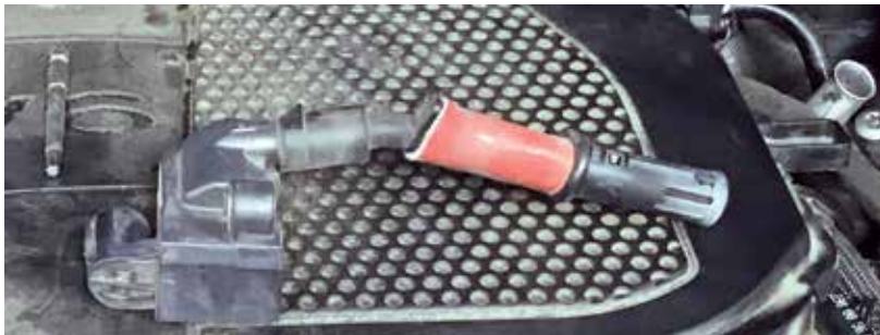
Note the white discoloration on the end of this COP boot. This could indicate spark leakage along the spark plug insulator to ground.
