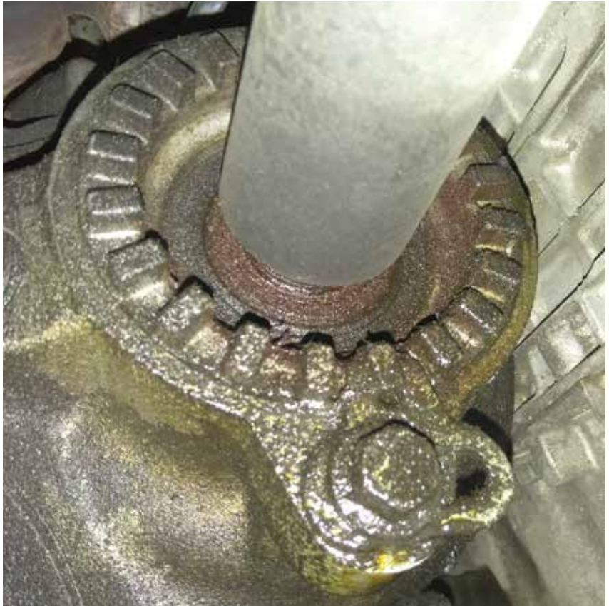
If you see gear oil leaking from the angle gear it should always be taken seriously, since Volvo's angle gears only hold about .85 quarts of gear oil when they are full. So it won't take much time for the angle gear to run dry.
