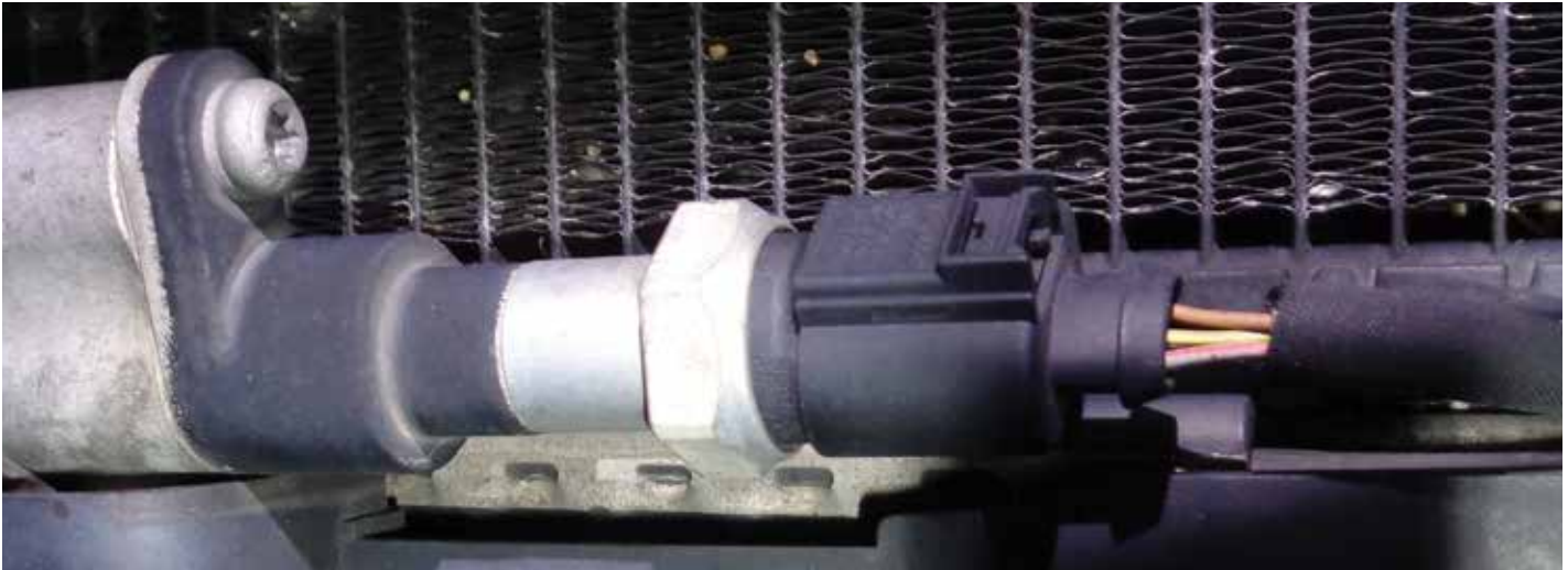
This sensor is readily visible through the front grille of most late model Audi vehicles. Always check this area if leaks are suspected.
