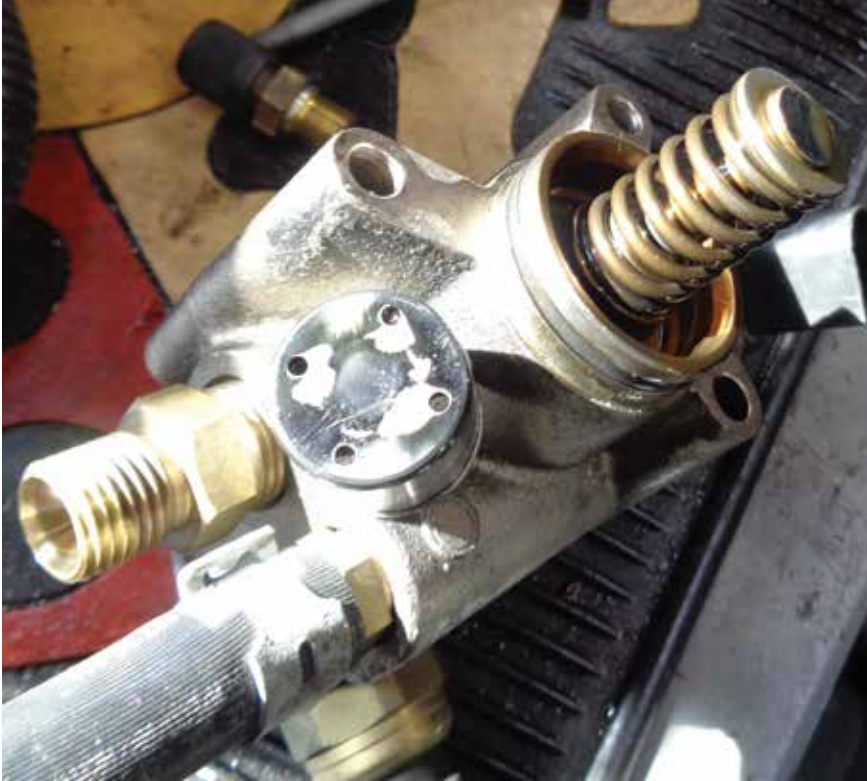
This high pressure fuel pump shows signs of wear on the piston head as well as cam follower. It should be replaced.
