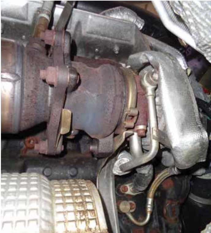
It may be necessary to heat stubborn exhaust hardware to aid in removal.
