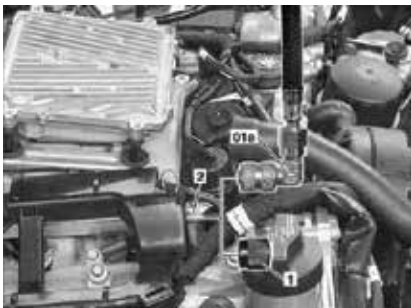
There's almost always a convenient Schrader on the rail for testing actual fuel pressure.
