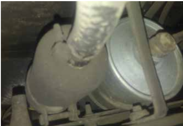
Main fuel pump
