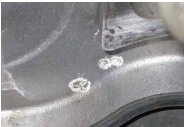
This is an example of corrosive action causing pitting in an aluminum housing.
