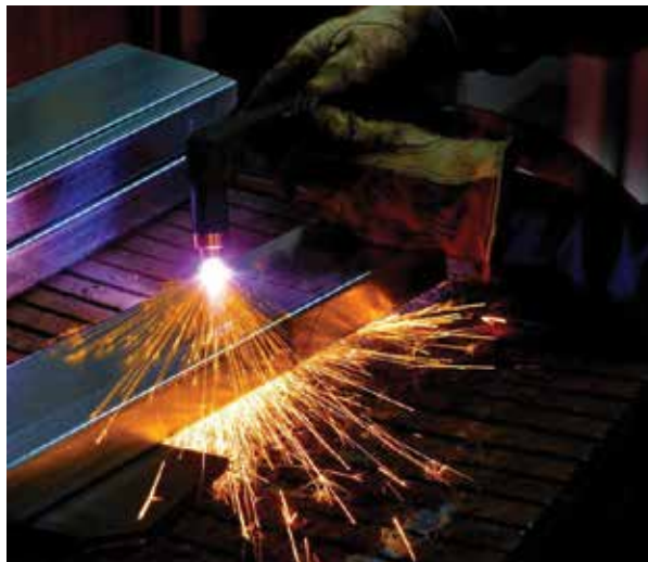
Great welds make solid repairs that usually are at least as strong as the sheet metal around them.
