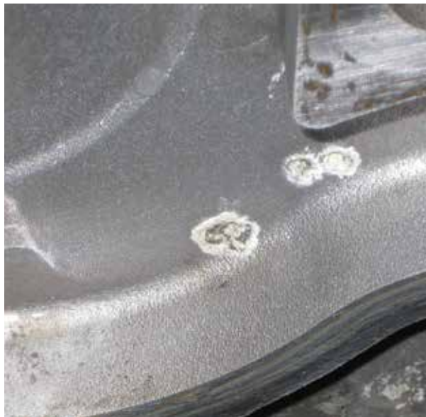
While the corrosion in this water pump housing is just getting started, in a short time it will grow and eventually impede the coolant flow. Genuine Mercedes-Benz antifreeze/anticorrosion protects against this.
