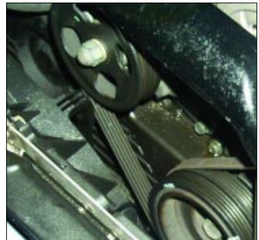
Drive Belt Inspection
