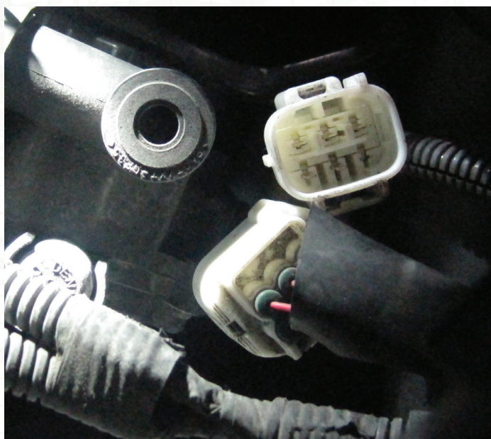
The three way valve has five circuits occupying a six pin connector.
