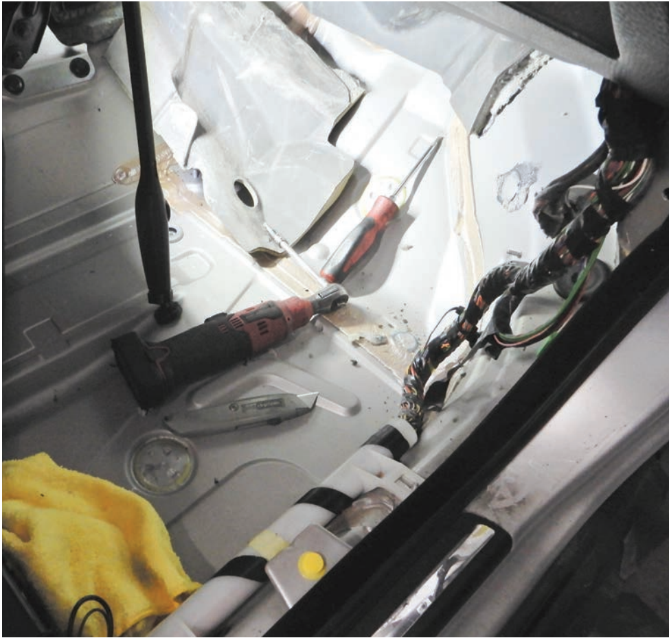
Cutting the soundproofing insulation around blower motor
