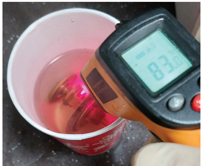
Testing the thermostat with hot water and a temperature gun
