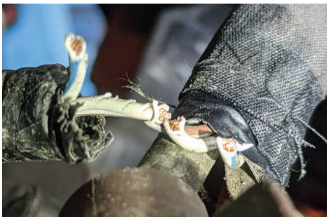
CAN wiring damage
